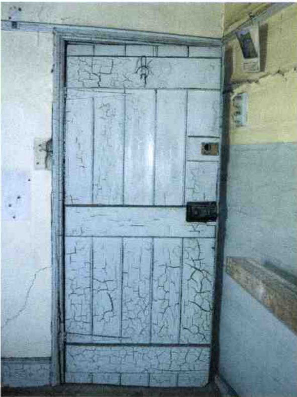
D39 rear face, ledged and braced door
