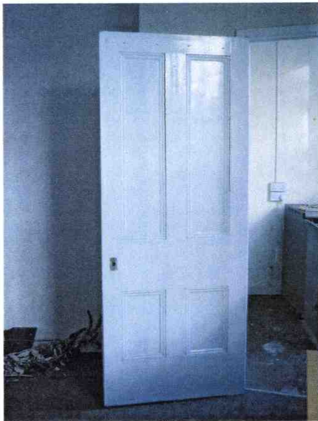
4. F2 office D3 to inner office F3.
