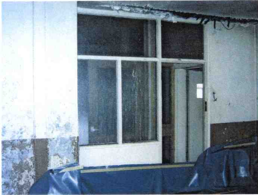
33. S5 Fire screen from landing S7. Polythene sheeting on floor.
