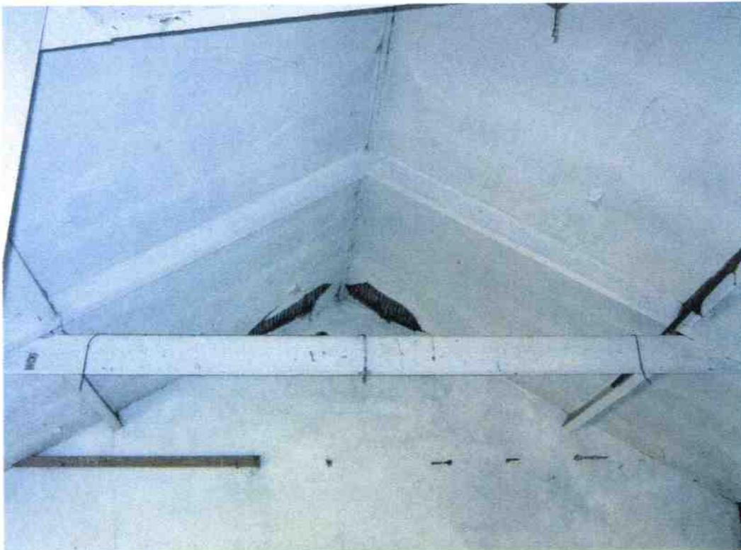
40. S8 Roof truss and collar – lath and plaster ceiling.
