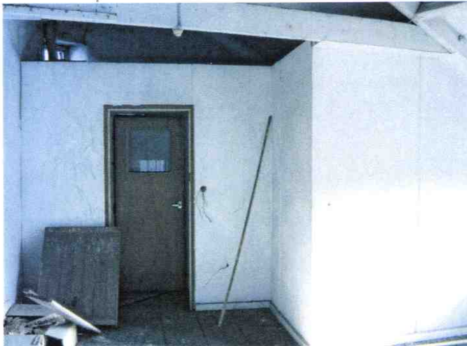
38. S8 Looking towards internal partitions to S9 and S10. D30 (open) in background.
