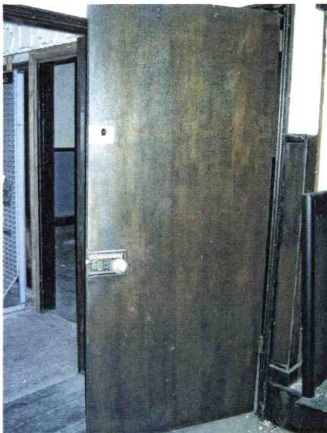
52. S16 D45 internal view. Varnished ply flush door.
