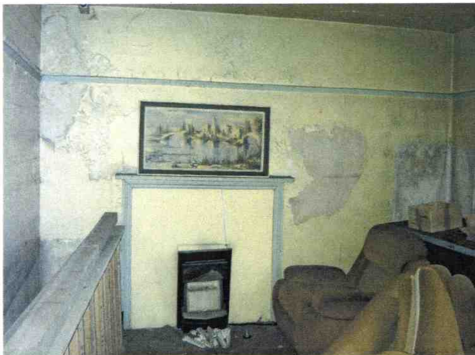
46. S14 Fire place and gas fire.
