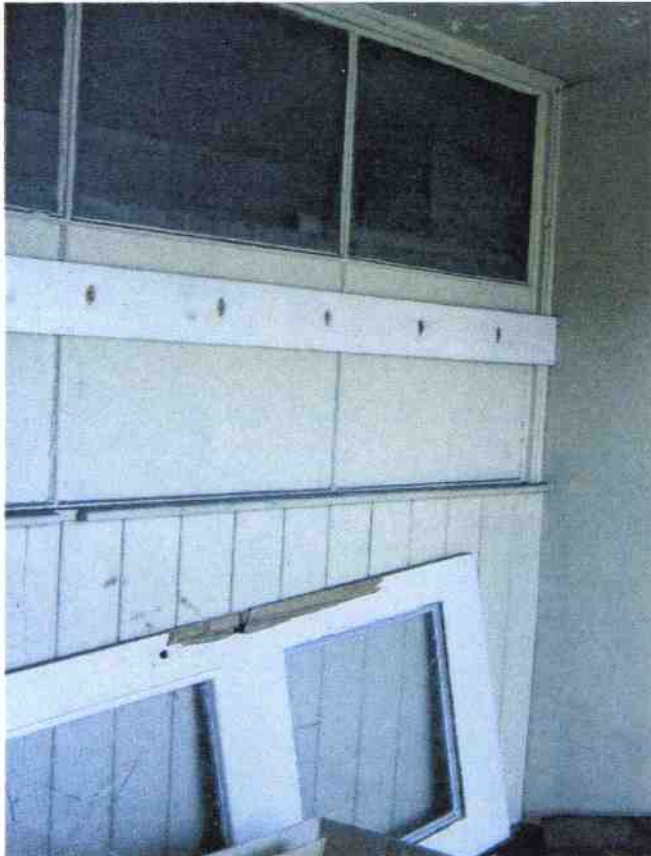
42. S12. Internal match board and glazed screen to S21
