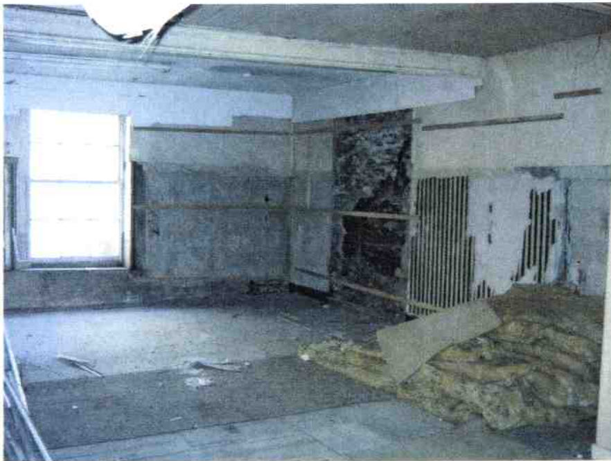
21. F17 Looking towards W10 + removed fireplace.
