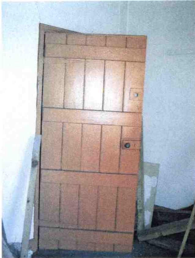
43. S13. Internal ledged and boarded door D38.
