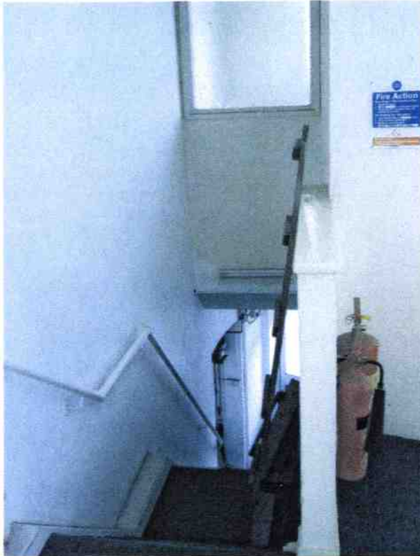
1. F1 First floor landing + staircase from street.
