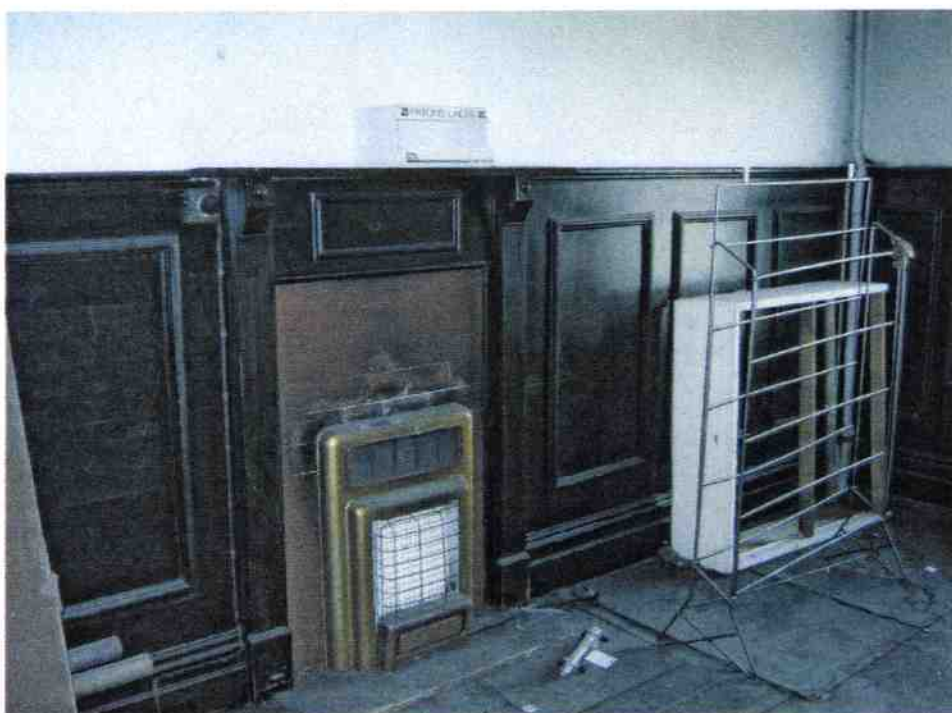
53. S16 Dado paneling (varnished ply) and gas fire.
