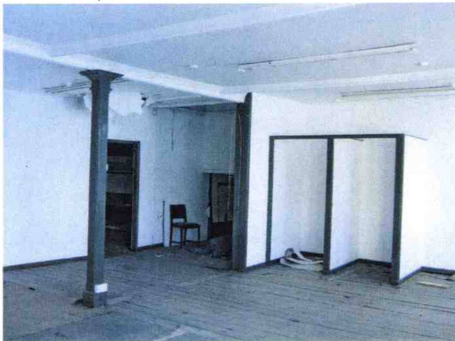
22. F17 Looking towards rear changing cubicles. Central support timber post.
