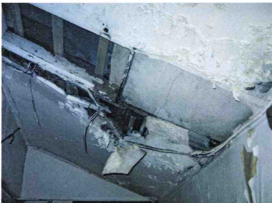
57. S18. Lean to roof – asbestos lining
