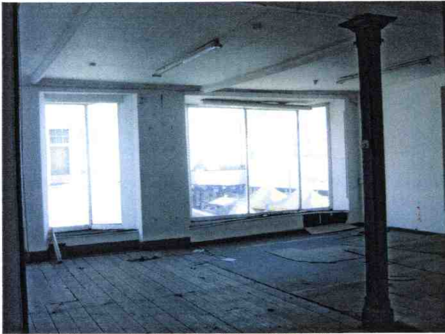
22. F17 Looking towards windows W12 + 13. Central support timber post.
