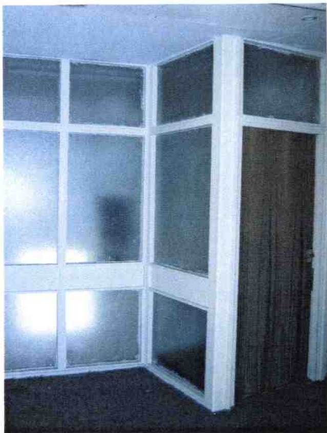
25. S1. Landing. Fire screen and D21.
