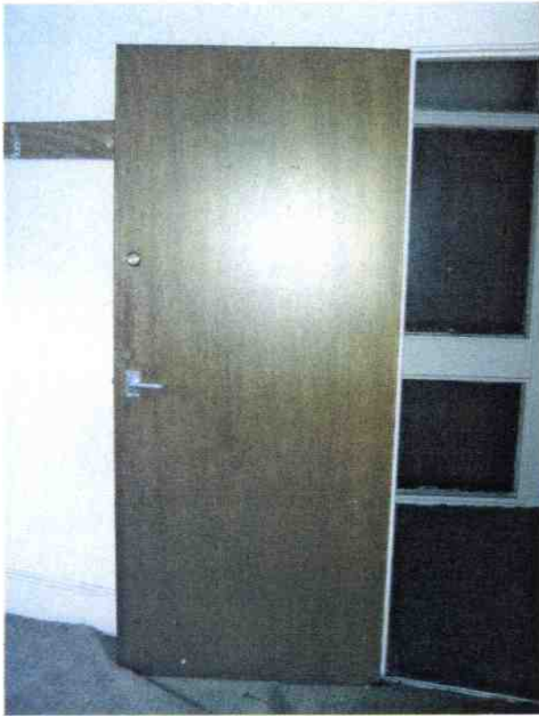
27. S4. D22. (Typical flush fire door)
