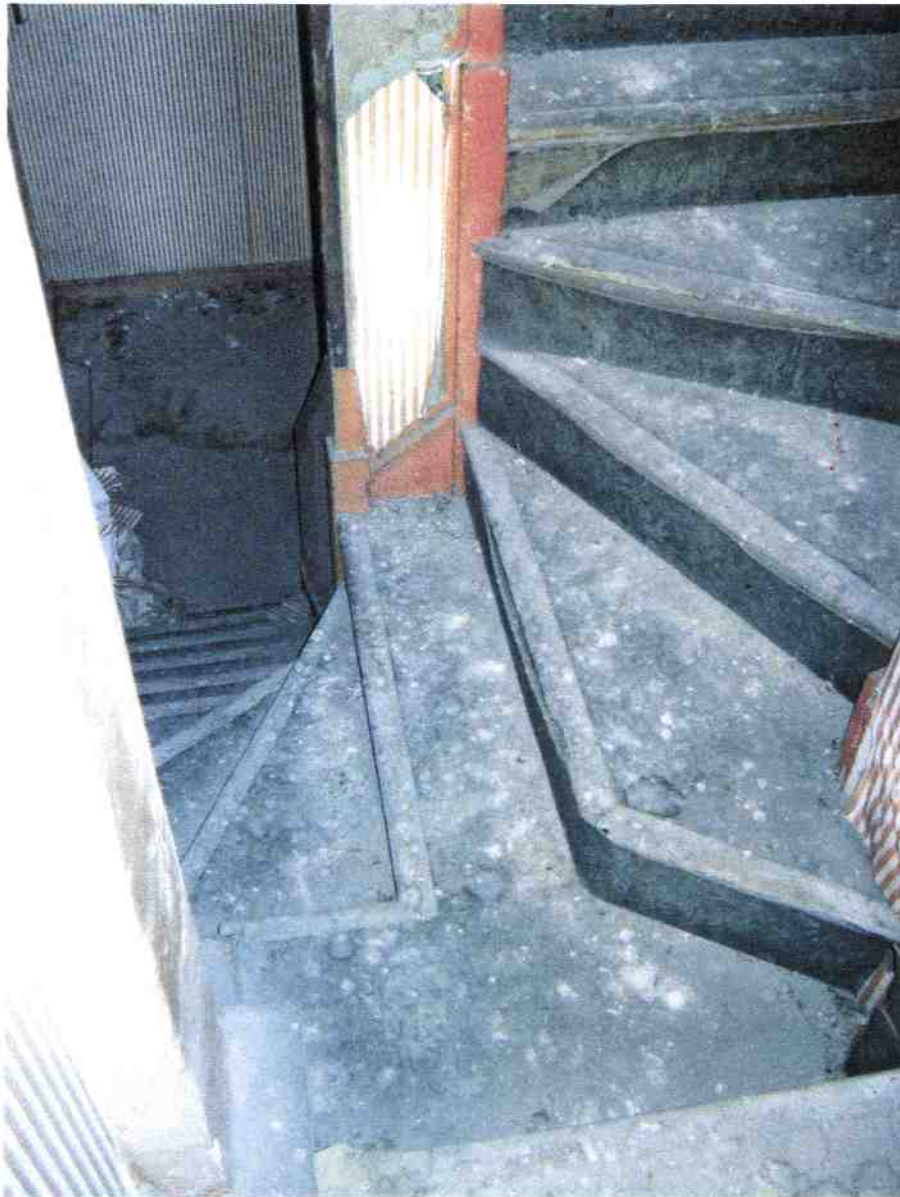
14. F7. Stairs at half landing.
