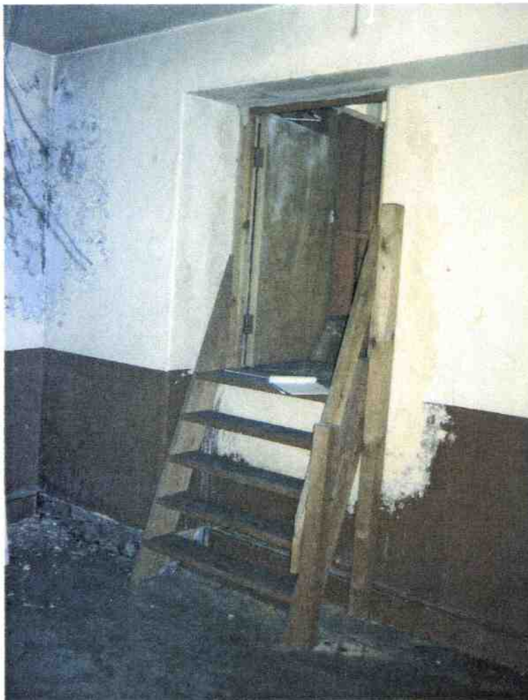
32. S5 Ladder to upper level (S8) + D33.
