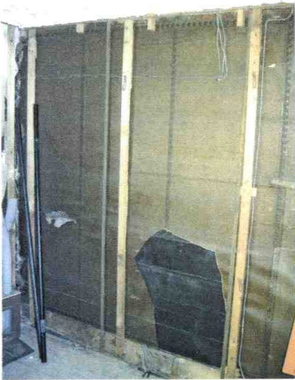
49. S15 View of part demolished partition and "leather" lining paper over timber boards.
