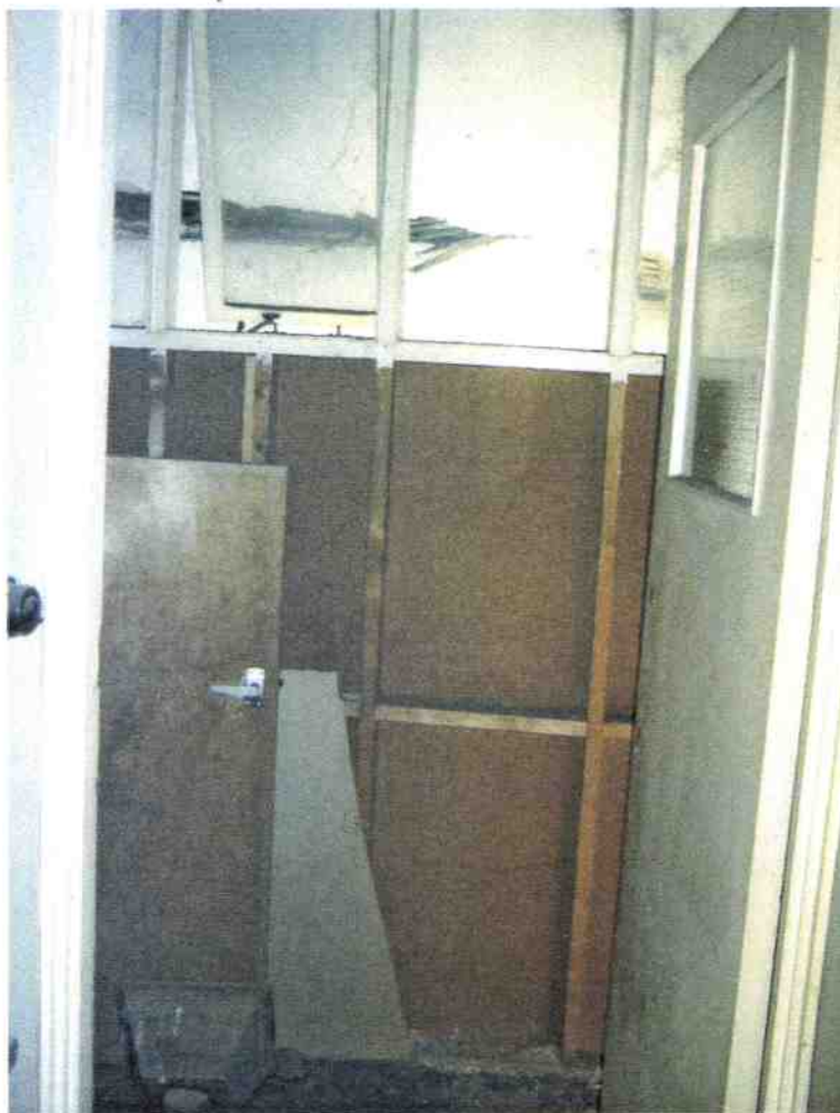
36. S9 D31 and internal hardboard partition.
