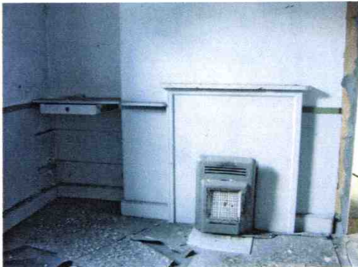
8. F5 fire place and gas fire.
