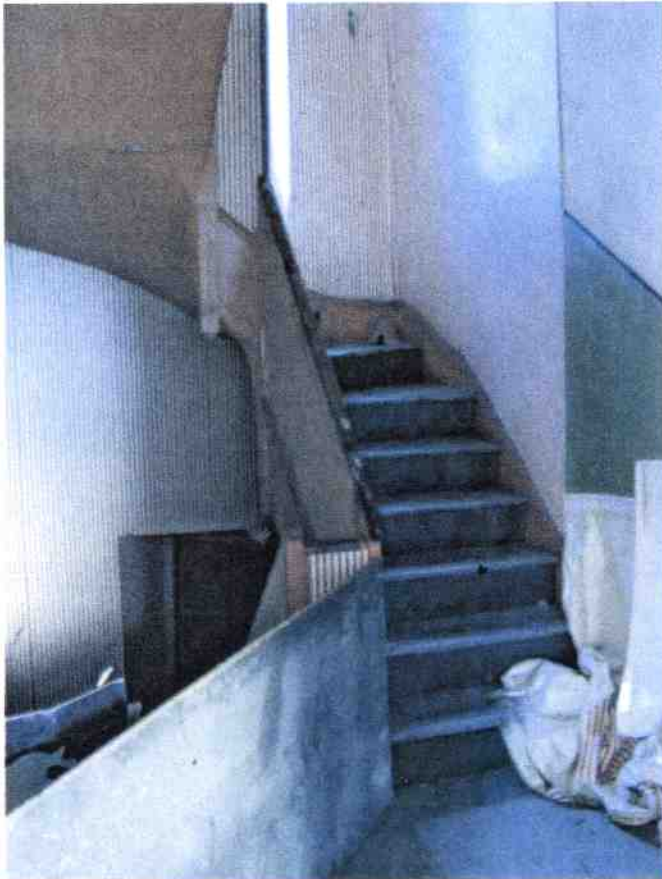
12. F7 landing, stairs to second floor.
