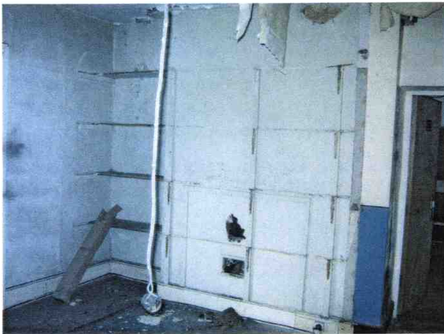
35. S6 Internal N fireplace wall + shelf brackets.
