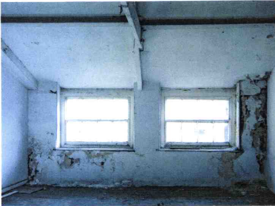
39. S8 W36 + W37. Lath and plaster ceiling.
